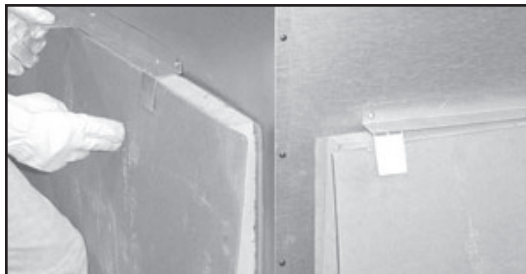
Figure 3.6 Unpacking Back Refractory
